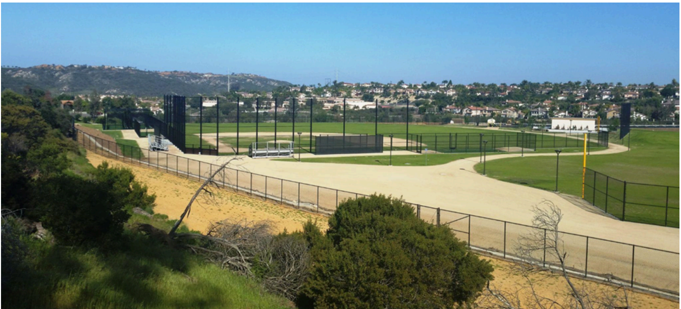
La Costa Valley Sports Complex Field
